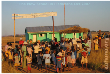
Community built school
