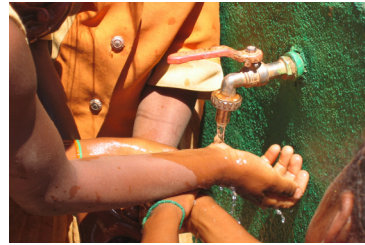
Community built water system
